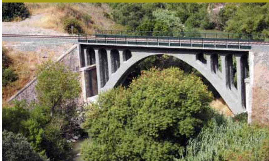
The first iron railway bridge over the Guadiaro as seen from the walk
