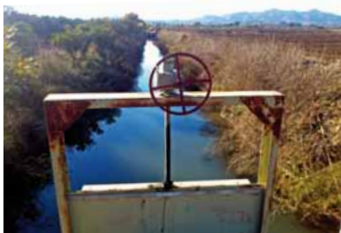
Main channel's sluice
