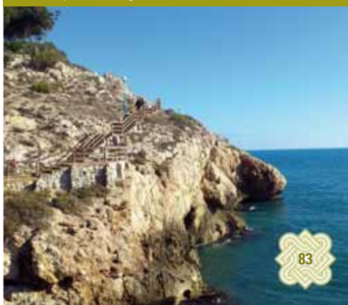
A walkway conditioning in El Cantal cliffs
