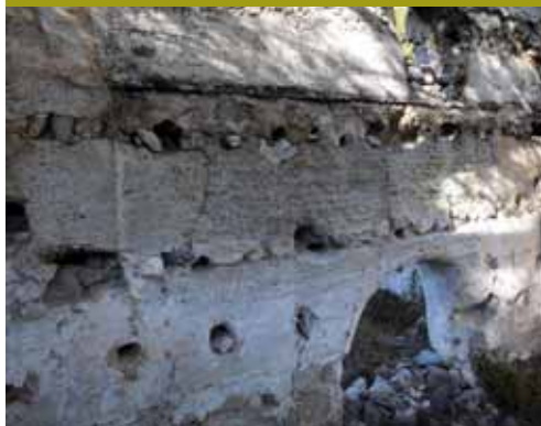
Layers of rammed-earth wall over an arch-shaped opening, Venta del Cebollero
