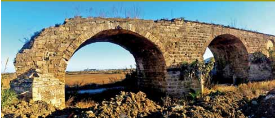
El Puente del Rey, unfinished construction destined to connect and provision the province capital
