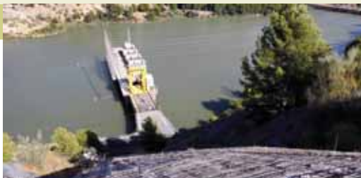
The back view of the penstock seen from a bend in the path, on a slope leading towards the Embalse de la Encantada
