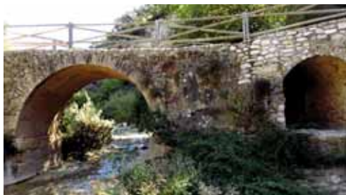
Bridge over the Río Burriana
