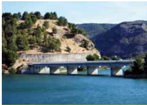
Bridge joining the Guadalhorce and Guadalteba reservoirs
