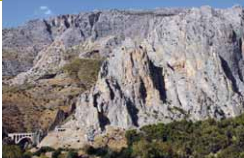
The cliffs known as Placas Frontales and one of the most beautiful railroad bridges
