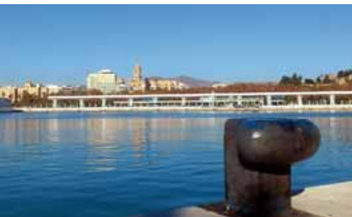
The Málaga Cathedral and the new boardwalk as seen from the port
