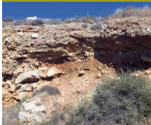
The embankment of the old railway line reveals the geological composition of the cliff
